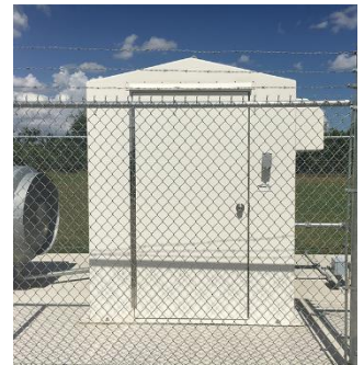
Shelter set up on site
